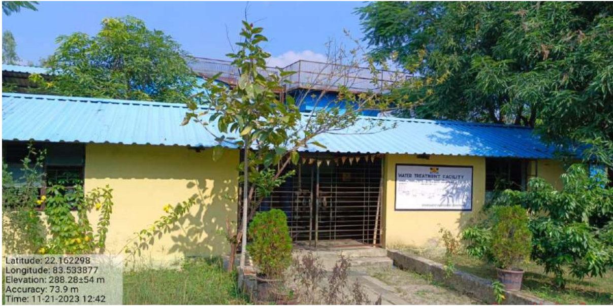
Reverse Osmosis Plant
